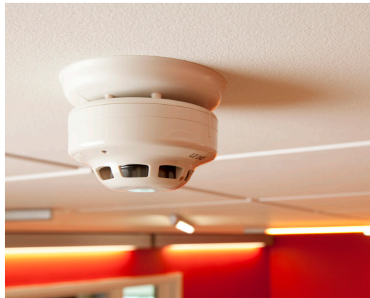
Fire alarm system
